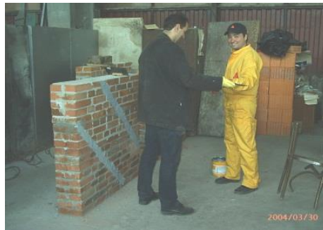
Image 1 Marking the position of the lamellas
