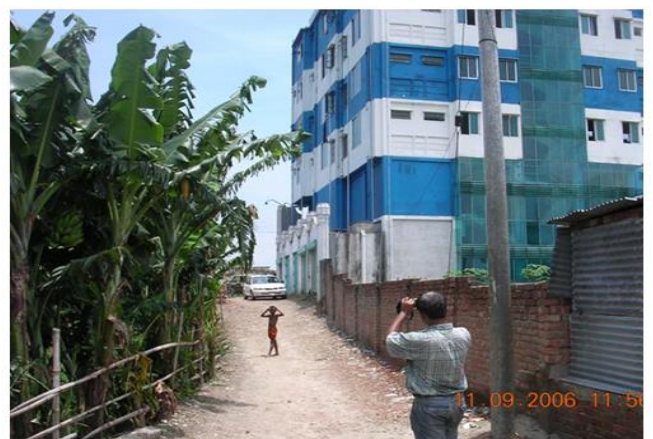
Figure 6: Photo was taken during road reconnaissance and field survey preparation, the Chowdhury Villa at Ch 1+550
