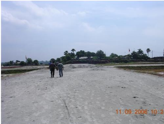
Figure 7: Photo was taken during road embankment at Kalshi Beribad at Ch 2+950
