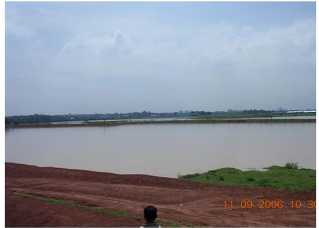
Figure 5: Photo was taken during road embankment preparation at Ch 4+050
