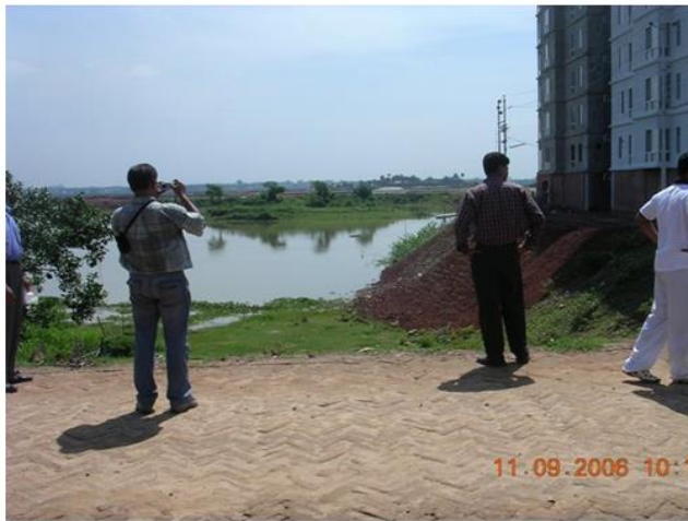
Figure 8: The endpoint of road, South-eastern corner, Source; project folder, the photo was taken during reconnaissance in 2006.
