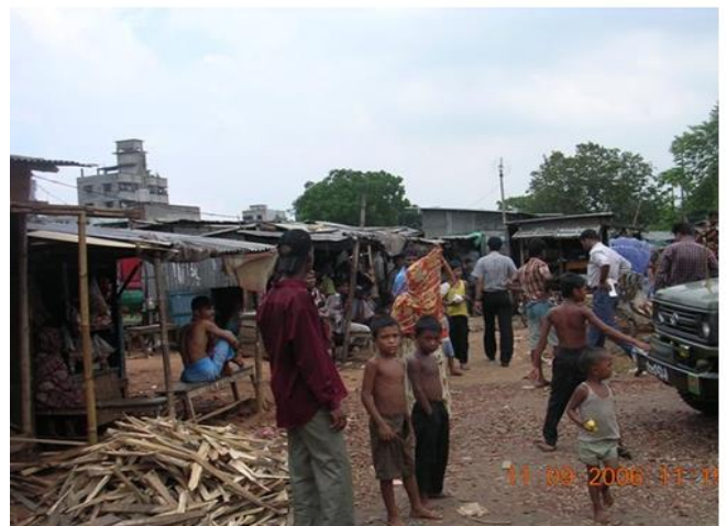
Figure 6: Photo was taken during road embankment preparation at Ch 4+050
