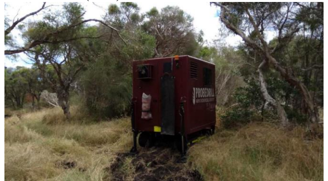
Figure 50: Photo 13: Conducting Cone Penetration Test at the location (CPTu1)
