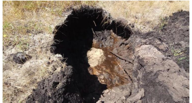
Figure 26: Soil Profile, Test Pit location (TP10) and ground watertable encountered at a depth of 0.7 m
