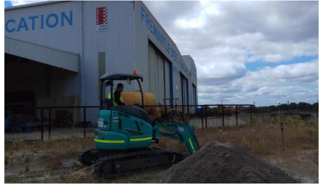
Figure 41: Photo 04: Subsurface probing by excavator at Test Pit location (TP1)
