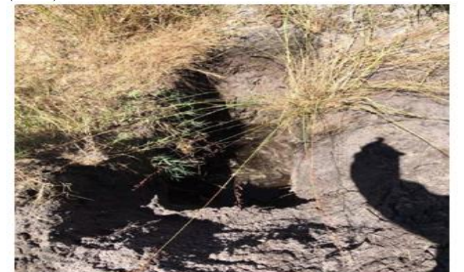
Figure 28: Soil Profile, Test Pit location (TP11) and ground watertable encountered at a depth of 0.9 m
