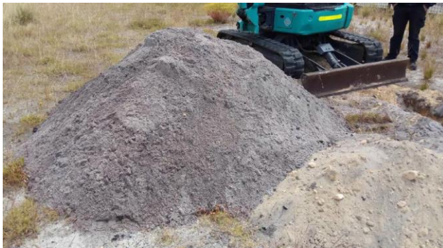
Figure 10: Soil from Test Pit location (TP1)
