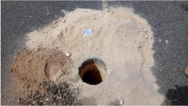
Figure 37: Spoil from Pavement Dipping 1 (PD1)
