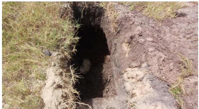
Figure 11: Soil Profile, Test Pit location (TP2) and ground watertable encountered at a depth of 1.8 m
