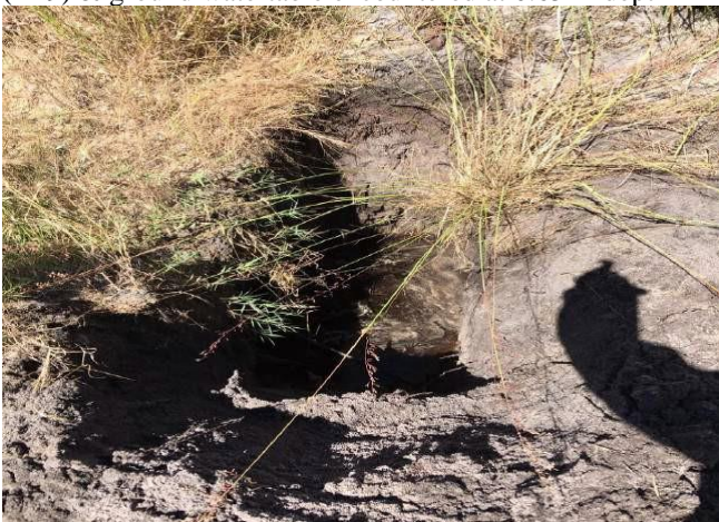
Figure 47: Photo 10: Soil collapsing into Test Pit location (TP11) & ground watertable encountered at 0.9 m depth
