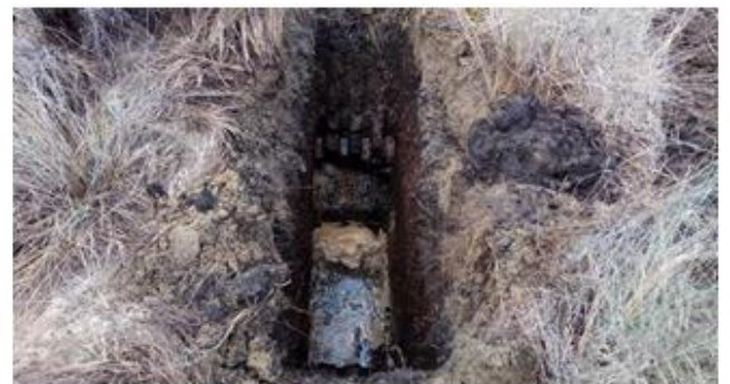
Figure 19: Soil Profile, Test Pit location (TP6) and ground watertable encountered at a depth of 1.2 m
