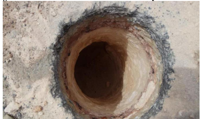
Figure 36: Pavement Profile of Dipping Location PD1
