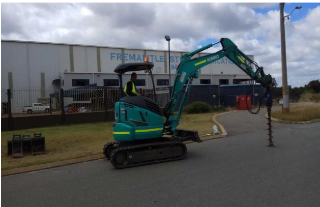
Figure 40: Photo 03: Pavement Dipping/drilling at the location (PD1)
