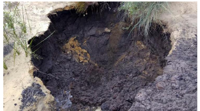
Figure 42: Photo 05: Soil collapsing into Test Pit location (TP3) and ground watertable encountered at 1.2 m depth
