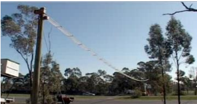
Figure 26: Rope net hooked between two poles, Possum and Fauna crossing (ladder type), Source: Nationwide Netmakers Pty Ltd
