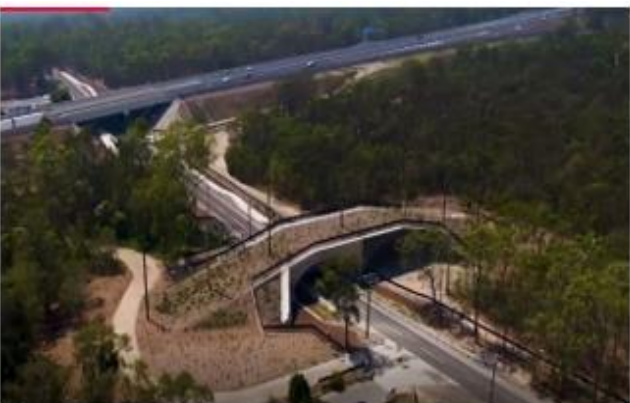
Figure 17: The Motory considered overpass and underpasses to mitigate these sensitive environmental impacts. Source: 9 News Adelaide; Ducks cross the road, 15 May 2019
