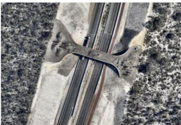
Figure 13: The newly build an overpass on Tonkin Highway in Ellenbrook, Source: NearMap image on 21 November 2020,
