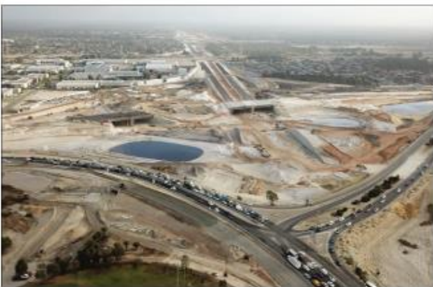
Figure 12: Tonkin Highway construction in Ellenbrook, Source: WAtoday, Hamish Hastie,
